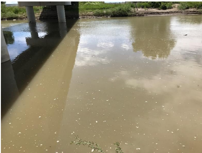
Photo 17. Across at Vaughn-Ulm Bridge Site.
