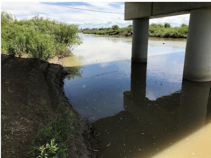
Photo 18. Downstream at Vaughn-Ulm Bridge Site.
