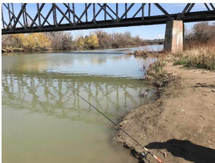
Photo 21. Downstream at Great Falls Site.
