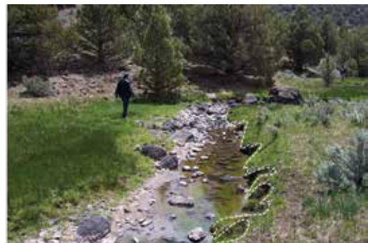
Figure 33. On this stream, the irregular bank margins (white dotted line on right bank) are evidence of lateral instability.
