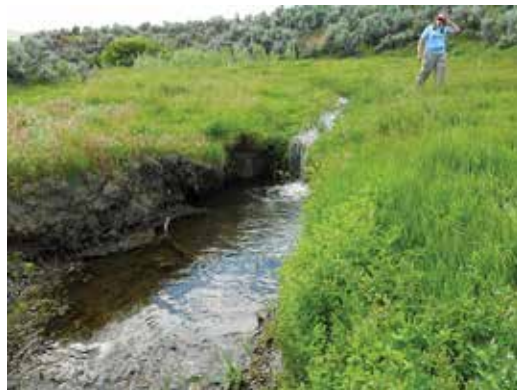
Figure 37. A headcut is moving upstream through a meadow, making the riparian area upstream of the headcut functional-at risk.
