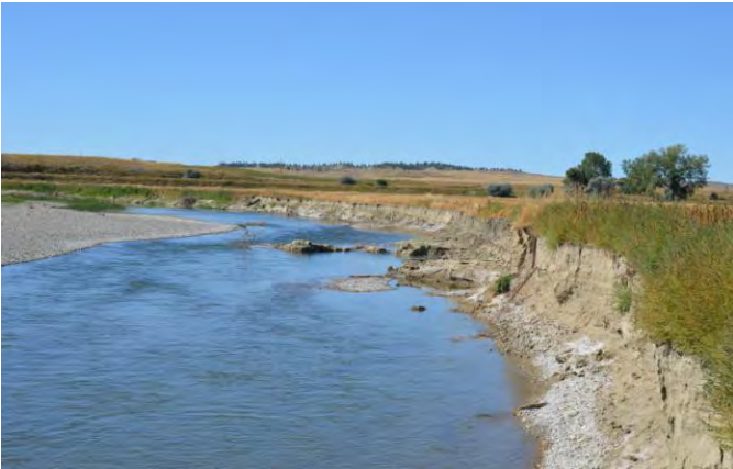
Moderate bank erosion occurring on isolated outside bends adjacent to hay field. Score = 3.
