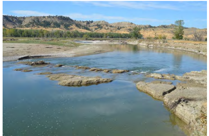
Visible scour of erosion resistant substrate layers may be an indication that entrenchment has occurred.
