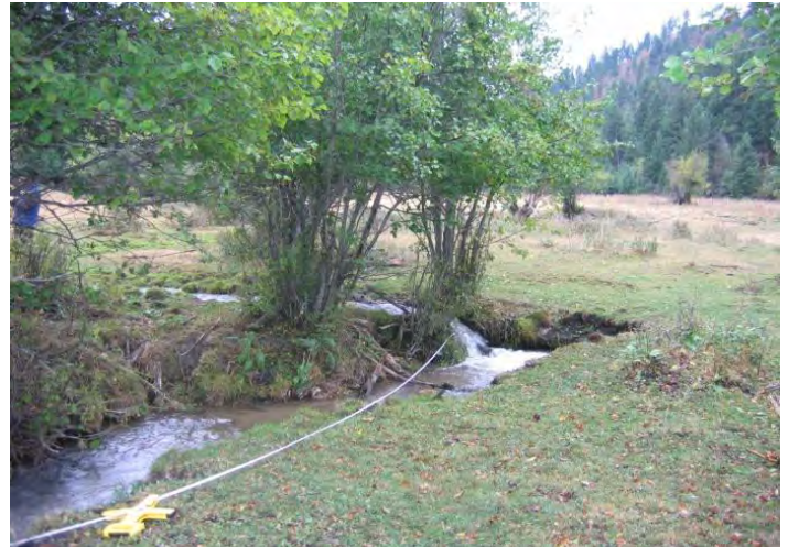
Small headcut in early stage. Immediate action may prevent further degradation. Early Stage 2 Schumm's model = Score 4.
