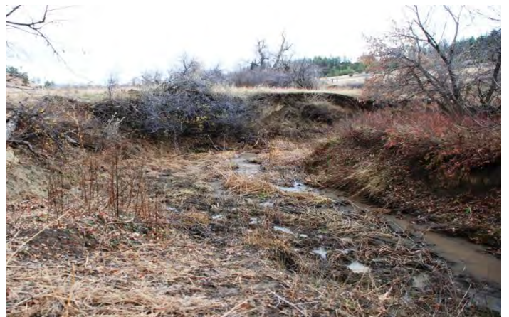
Channel has begun stabilizing. Vegetation establishing at base of banks. Stage 4 Schumm's Model = Score 6.
