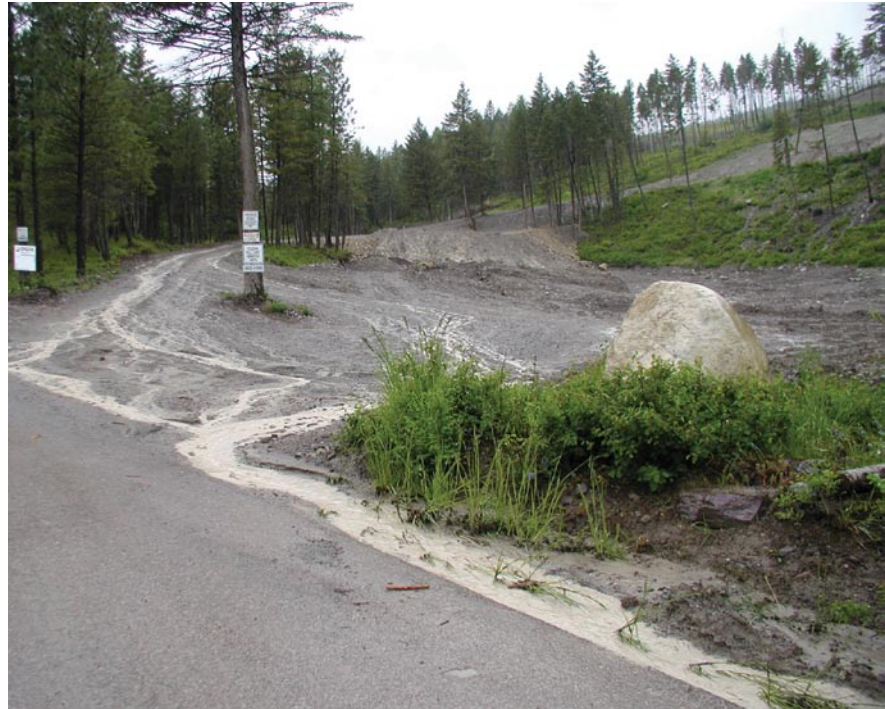
Poor road design can increase sediment loads to local water bodies.
