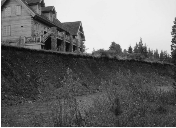
This home was built out of the floodplain—but on an erosive bank overlooking the Shields River. In areas where streams are known to meander, building setbacks and vegetated buffers should incorporate non-floodplain areas overlooking the stream—because as valley stream channels naturally meander, these homes can become vulnerable to falling into the water.
